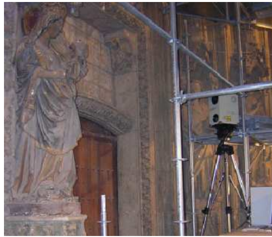
Figure 1: Scanning process on the scaffolding of the portico.
